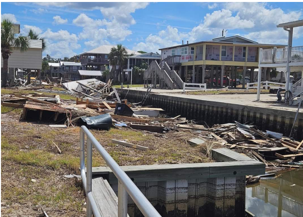
Damage caused by Hurricane Idalia
